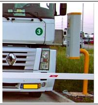
Ticket printer and information machine – placed at the barrier, easy to handle, can be accessed from a truck as well (elevated)
